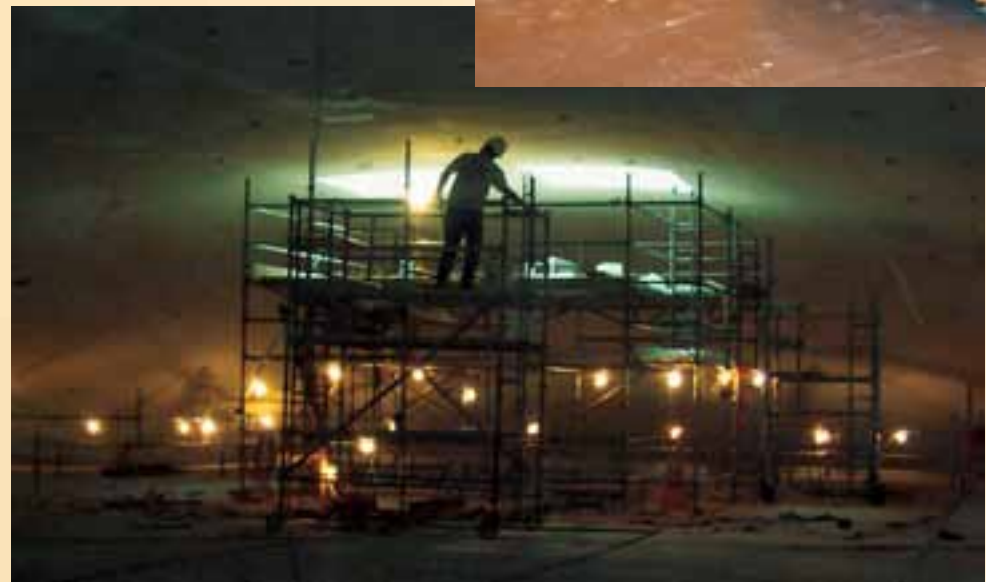
A worker stands atop scaffolding that is several stories high as he works on the restoration of the ceiling. Fourteen layers of paint were removed to reach the original plaster. After repairs were made, workers applied plaster that matched the properties of the historic plaster in both its content and acoustic properties. Care was taken to preserve the waviness of the original ceiling.
