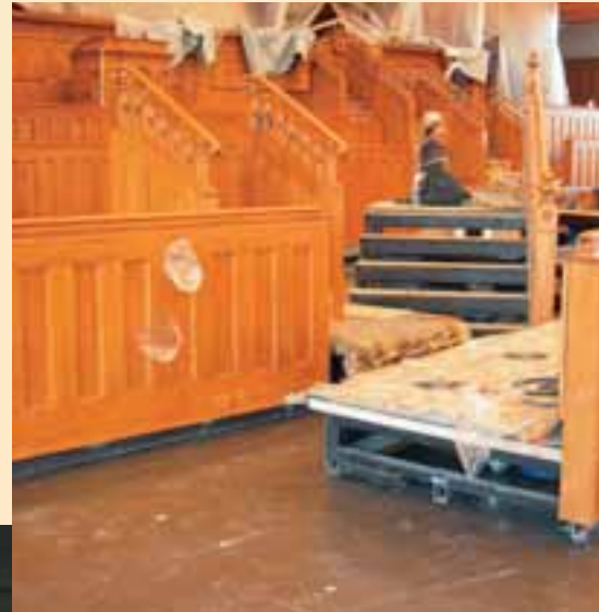
Right: The rostrum has been equipped with a large stage lift in the center. This, in combination with self-contained rostrum wagons (right), can be configured into general conference mode, fireside mode, or orchestra platform mode. The wagons have audiovisual equipment, wiring, and ventilation built into them. They also have matching carpet, new millwork, and viewing screens on which General Authorities can watch conference proceedings.
