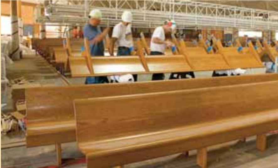
Above: Workers install solid white oak pews , which will replace most of the original soft pine ones. The original pews, painted by pioneer artisans to look like oak, were damaged and worn. Some will be permanently displayed.
