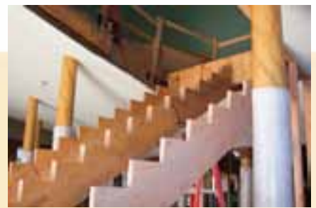
One of two new staircases added to the balcony makes six exits from the upper floor.
