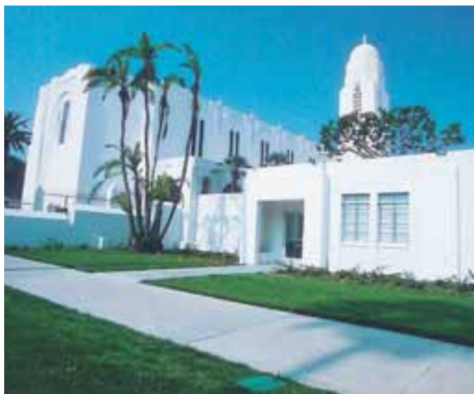
Originally dedicated in 1929 by President Heber J. Grant, the Los Angeles Stake Center was rededicated by President Gordon B. Hinckley in June after extensive remodeling.
