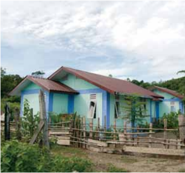
Yards have already been enclosed around these two of the more than 900 new homes built in Indonesia.
