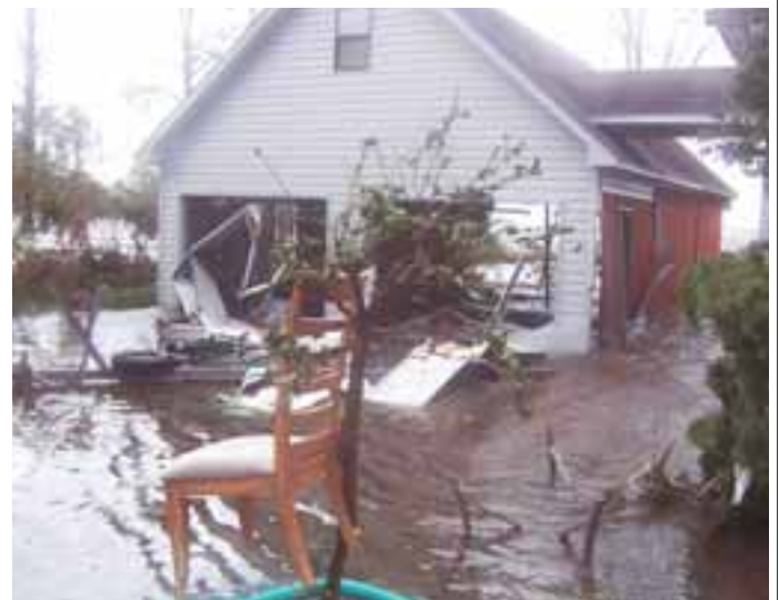
Wind and waves from the hurricanes destroyed many structures, including part of this home in Florida.
