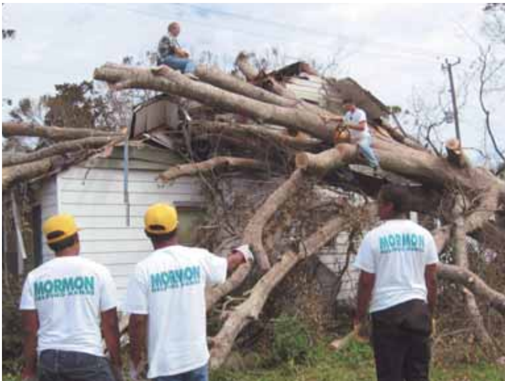
Latter-day Saint volunteers help remove a tree that damaged this home in Florida.
