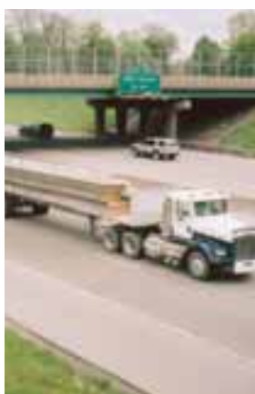
The location on Interstate 64 where the first East St. Louis chapel once stood.
