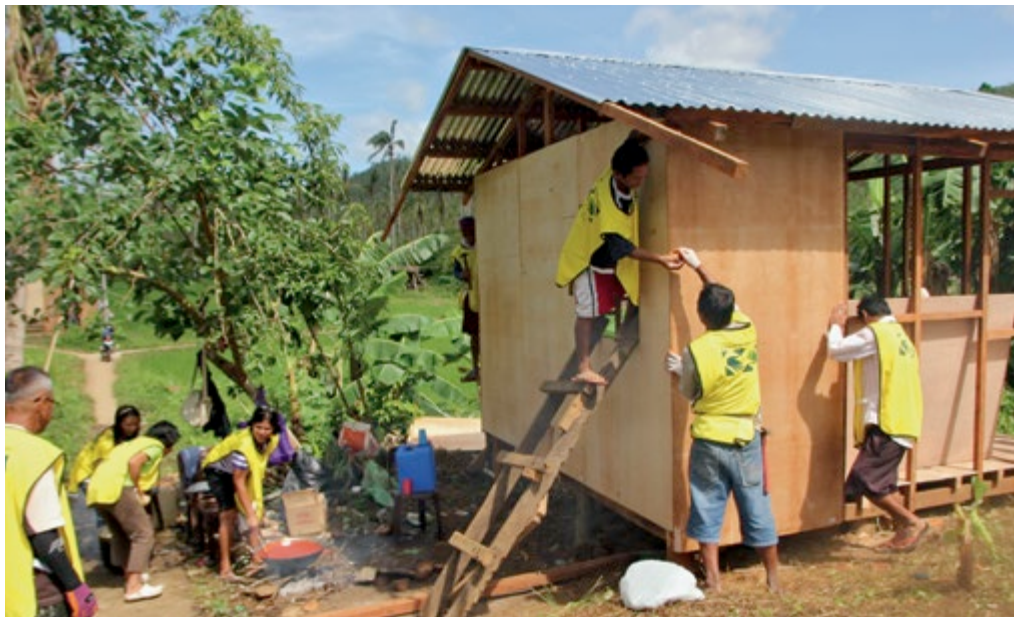
Volunteers nail plywood to the frame of a new house in Tacloban, Philippines.
