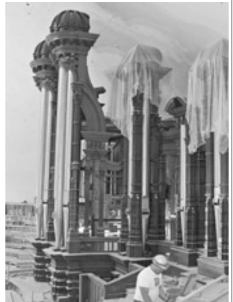
New gold leafing was applied to visible organ pipes.
