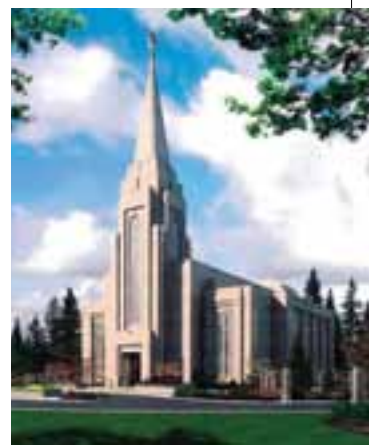
Ground was broken for the Vancouver British Columbia Temple on August 4, 2007.
