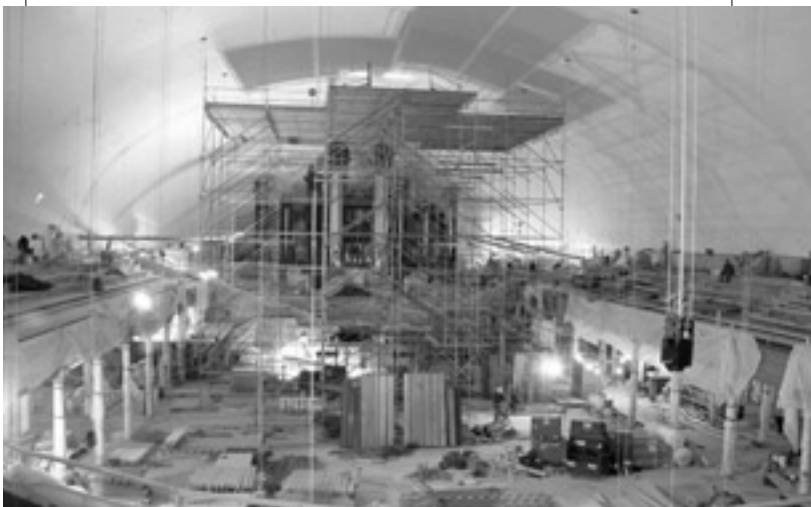
Renovation of the Tabernacle's interior included repairs to the ceiling, new seating, and the creation of an interchangeable rostrum and stage area.
