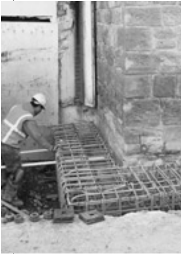
Seismic upgrades included a reinforced foundation.
