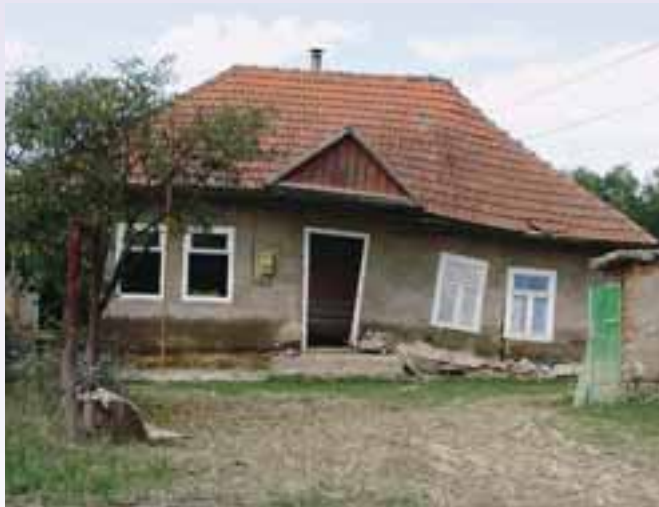
This home was one of 90,000 damaged by historic flooding in Eastern Europe.
