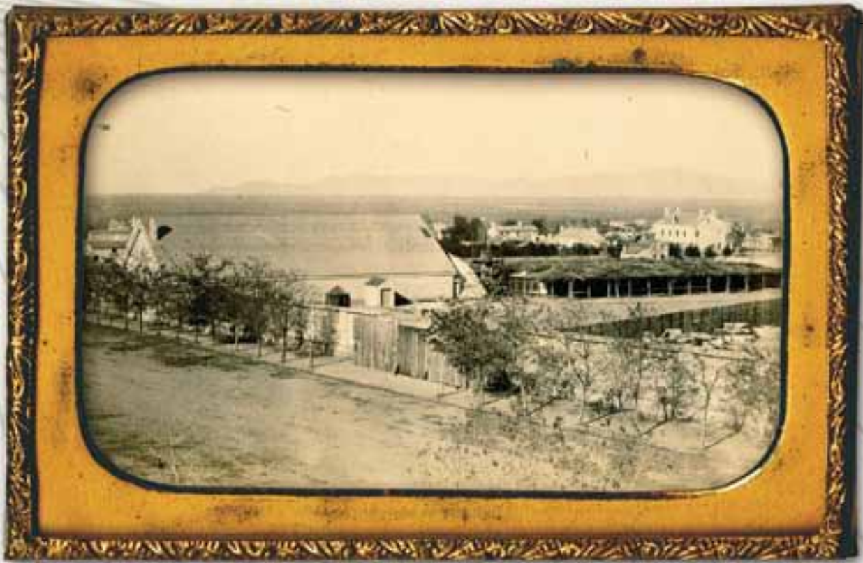
The first meeting place on Temple Square was the bowery, a simple pole structure with open sides and roofed with willow branches. This 1862 photo shows a later bowery, behind the Old Adobe Tabernacle. This bowery was enlarged as needed to
