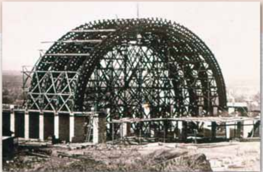
Above: The trusses were framed and put together on the ground and temporarily pinned. When everything was properly fitted and marked, the timbers were taken apart and raised plank by plank and put into place over scaffolding erected for that purpose.
