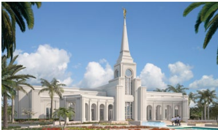
Ground has been broken for the Fort Lauderdale Florida Temple.
